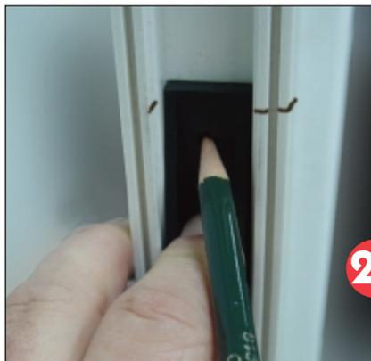
Open door, relocate Lock Catch to line up with pencil and mark holes (see Picture #21). Install Lock Catch using 1/4" self-tapping screws provided in Poly Bag #2. (see Picture #22) Use Spacer if needed. Lock Catch has slotted holes for adjustment if necessary.
