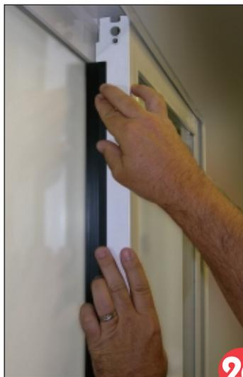
The Draft•Stopper™ attaches to the moving section of your sliding glass door. To install the Draft•Stopper™, measure the vertical distance, or height of exposed glass, between top and bottom frames of the sliding door. Cut Draft•Stopper™ to size with scissors using this length.
