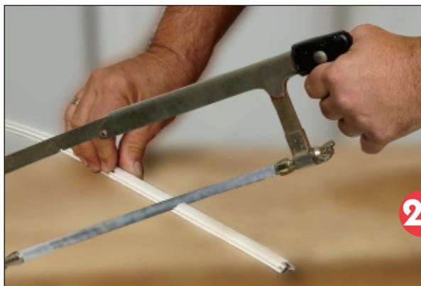
After measuring length, use a hacksaw to cut door Seal Extrusions to length (see Picture #24) and press into slots. (see Picture #25)
