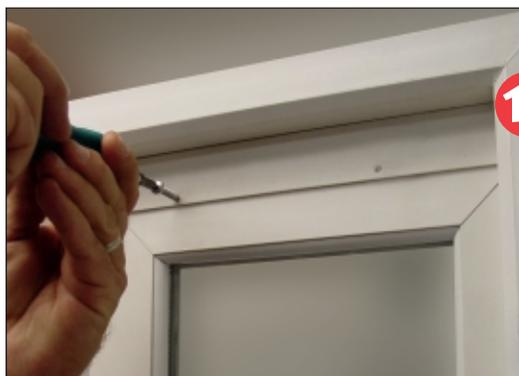
**WARNING: SCREWS PROVIDED ARE SELF-TAPPING, NO DRILLING REQUIRED. DO NOT USE DRILL BITS IN ANY PART OF THIS INSTALLATION.**
