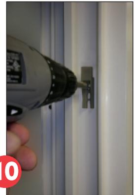
Using screws provided in Poly Bag #1, attach the hanger to the frame, keeping the hanger centered on frame (see Picture #10).
