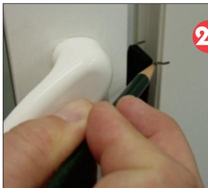
Partially close your sliding door so that you can mark the location of the top edge of Lock Catch inside your pet door frame. (see Picture #20)
