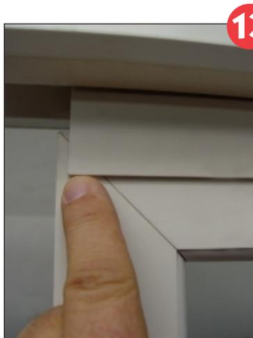
A gap of 1/4" must be left at sliding door-side area of filler section (see Picture #13) to clear the Door Seal Extrusion pieces.
